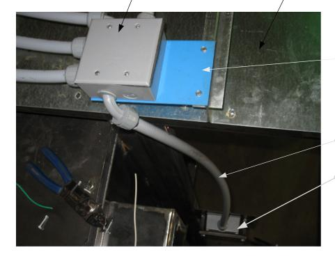
This box is secured to the panels by 2 screws.
