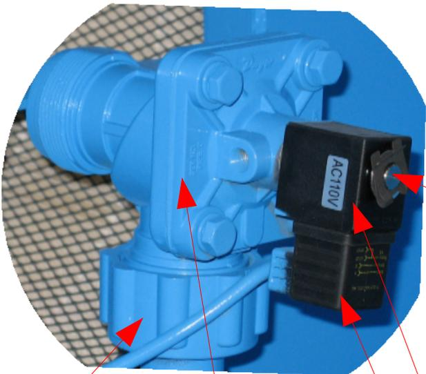
Valve to release air into the filters to clean them
